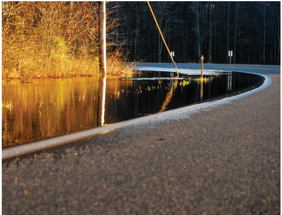
Flooded roadside in Dorchester County Courtesy of the Chesapeake Bay Program; photographer Matt Rath
