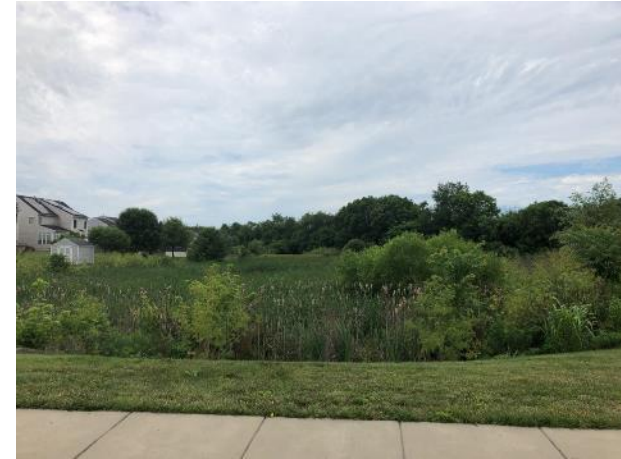
Bioretention Facility, Solar Drive
